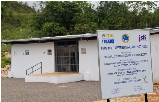
Water Valley Grading, Packing and Cold Storage Facility, which will directly benefit 100 farmers
